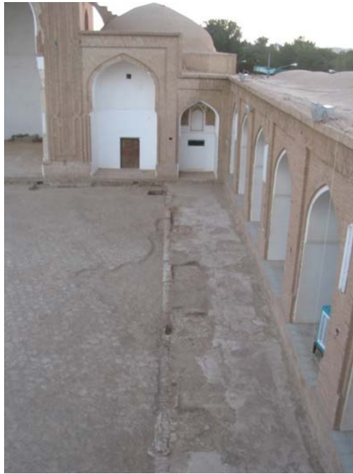
Fig .10. Discovery of the Original Peripheral of the Courtyard to the North Side, after ICHHTO
